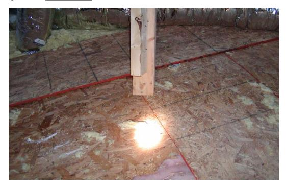
Improper support of purling, brace is not attached.
