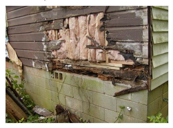
This repair was incorrect due to the non pressure treated wood coming in contact with concrete blocks, plus the floor has not support on the outer edges. There should have been an outer floor sill made of pressure treated wood.
