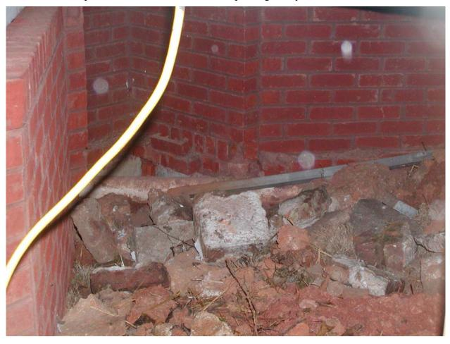
Fill dirt should be placed under porch and sloped away from structure.
