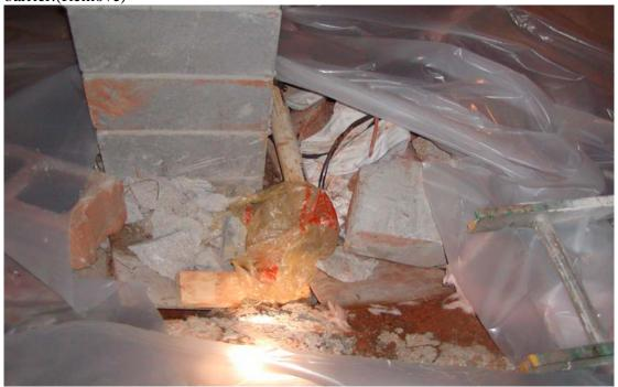
Girder has inadequate support at the end spans where Girder butts up against the wall.
