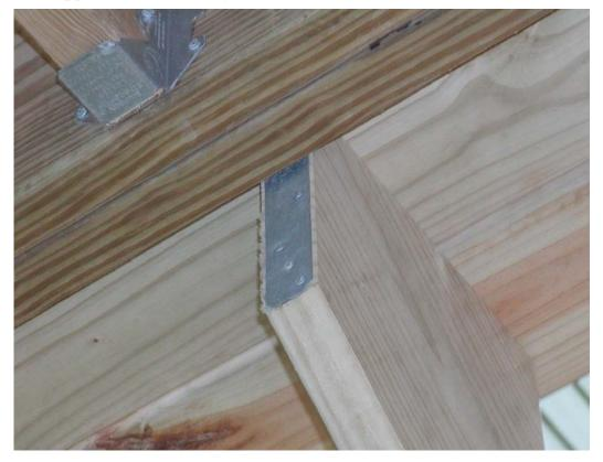
The proper type of joist hanger or stringer attachment should be, Simpson Strong Tie (LSU 26).
