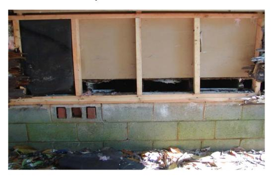
Part of the root cause of all of this wood decay under vinyl siding is improperly installed asphalt roof shingles. There was no starter shingle used which allows rain water to flow between the tabs and penetrate the vinyl siding which was not properly installed either.
