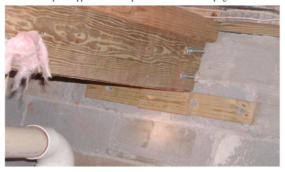
This method of framing is unacceptable. One end is supported by 2x4 blocks that are mechanically attached to foundation wall.
