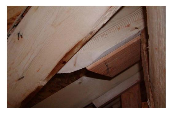
D) Rafter is cut to allow a vent from the water heater to pass through.
