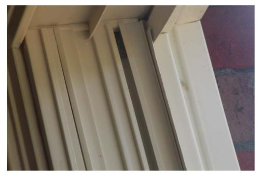
Side wall flashing is missing.
