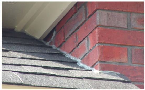
**§RR905.2.8.4 Sidewall flashing.** Flashing against a vertical sidewall shall be by the step-flashing method.
