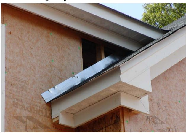
Brick veneer not properly supported by roof construction, additional rafters should be added.
