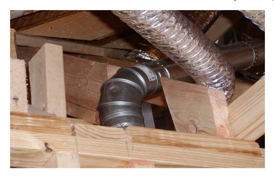
Poor installation of top plates and fastening.
