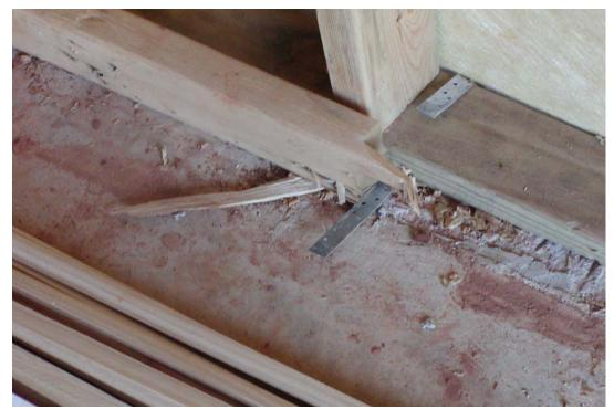
Low voltage wire is routed on the underside of floor joist. Re-route to avoid damage in next phase of construction schedule.
